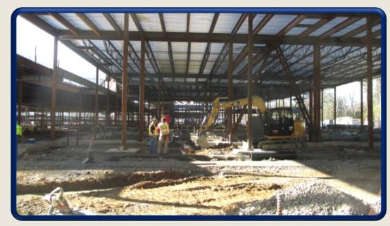
April 13th View of Area G – Facing West First concrete slab placement. Lower level roof (Green Roof Area)
