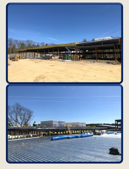
April 23rd View of Area A & B – 2<sup>nd</sup> Floor Metal deck prepped and reinforced for slab on deck placement. Placement scheduled for 4/25
