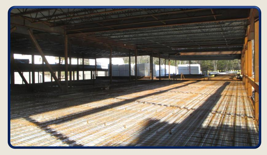
April 23rd View of Area A & B – East Elevation Exterior CMU masonry back-up walls in progress.
