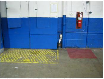
Fill port associated with the former 1,000 gallon waste oil UST located on west wall of automotive garage.
