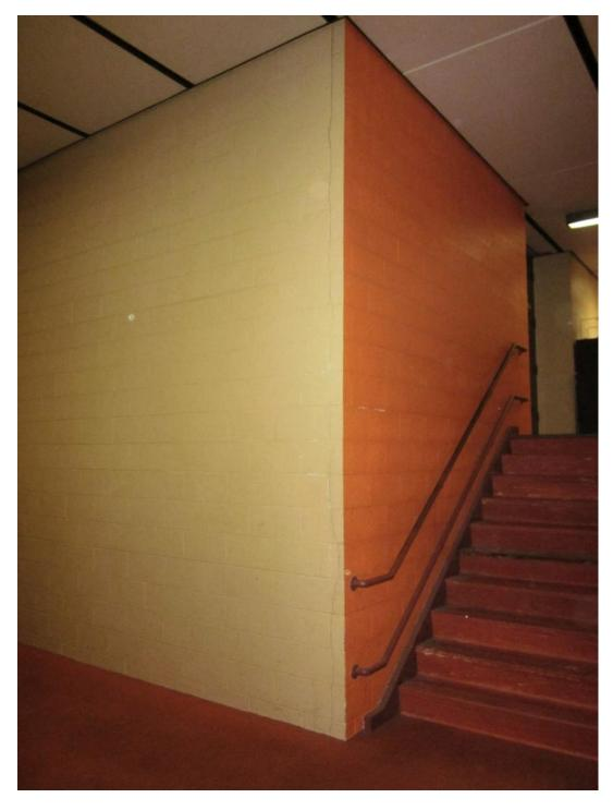
This photo shows another of the many locations throughout the school building where the interior masonry block partition walls are cracked.
