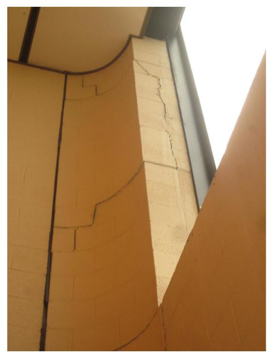
This photo shows the cracking and displacements of the masonry pier along the window of the multi-story stair towers at the east and west ends of the school building.
