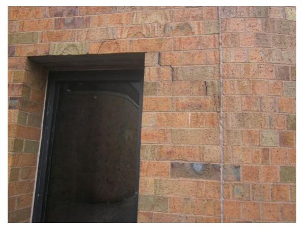
This photo shows one of the locations where minor cracking of the exterior brick veneer has occurred.
