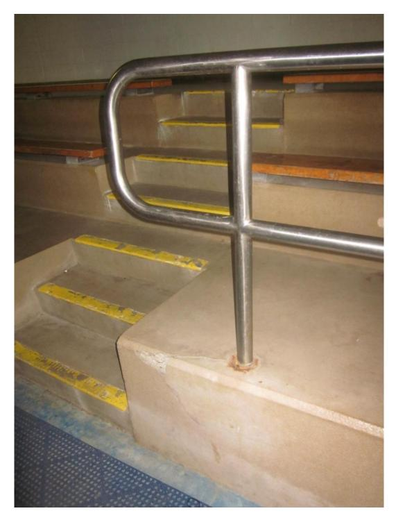
This photo shows one of the several locations where cracks and spalls have occurred where the natatorium bleacher seating guardrails are pocketed in the concrete.
