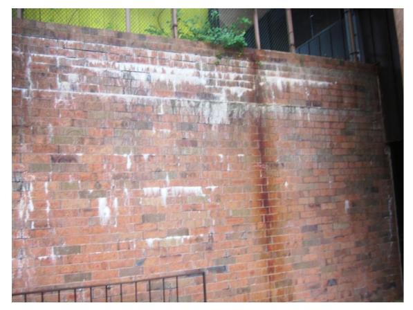
This photo shows the efflorescence leaching from the exterior brick walls along the east side of the Boiler Room building resulting from water infiltrating these walls from the terrace above.
