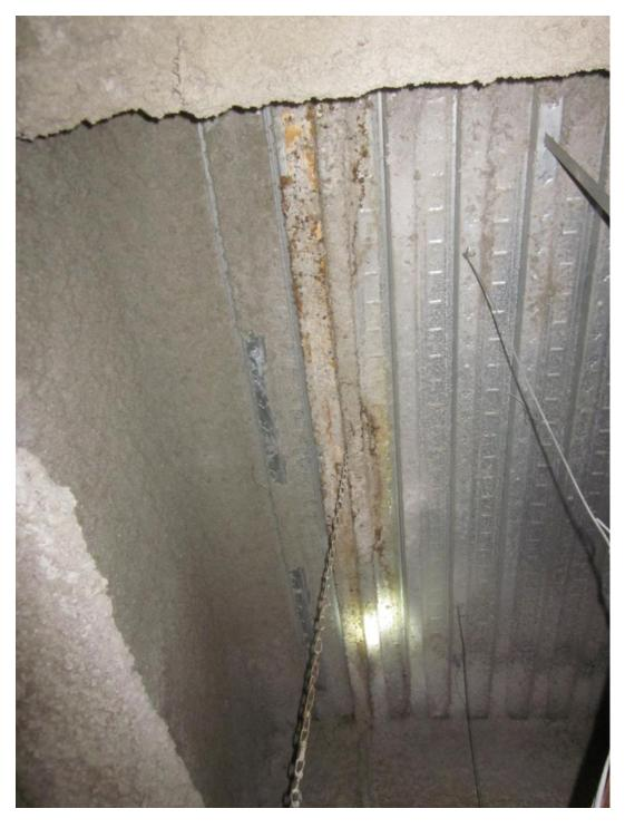
This photo shows the corrosion of the composite metal roof decking along one of the expansion joints in the roof of the school building.
