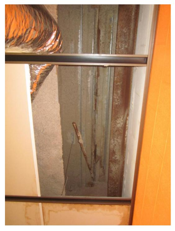
This photo shows another of the roof leaks that has occurred along the expansion joint adjacent to the Instructional Media Center.
