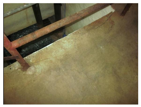
This photo shows some of the cracks and spalls in the natatorium and pool filter room concrete floor slab.
