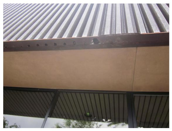
This photo shows the deterioration of the bottom closure plate at the base of the Cor-Ten metal siding on the west side of the school building.
