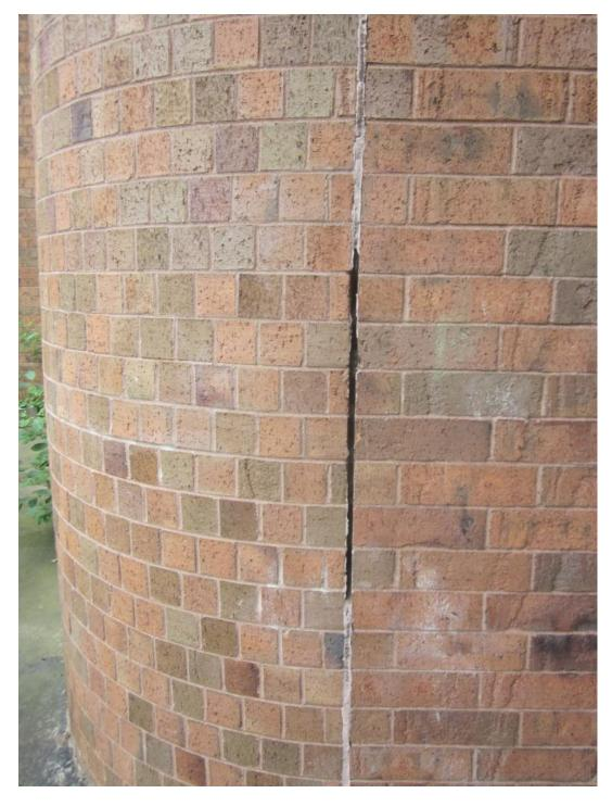
This photo shows another location where the sealant in the exterior brick wall control joint is missing.
