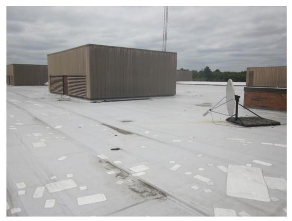
This photo shows some of the many patches in the aged roofing system on the school building roof.
