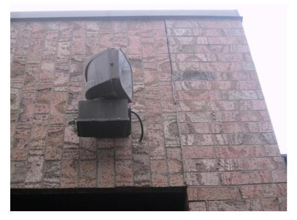
This photo shows another location where the sealant is missing from the top of the control joint, and the sealant is being squeezed out from the lower portion of the exterior brick veneer control joint.
