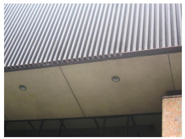
This photo shows a location where the bottom closure plate for the exterior wall metal siding panels was reportedly removed due to significant deterioration of the closure plate.
