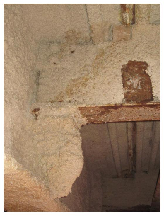
This photo shows the sliding-bearing assembly located along the east expansion joint of the multi-story building. Note the lack of the bent plate and the installation of the metal roof decking between the roof girder and the joint.
